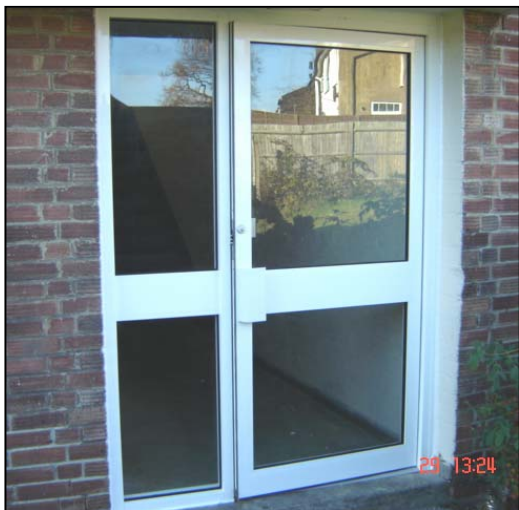
New security door at Shaftesbury Circle
